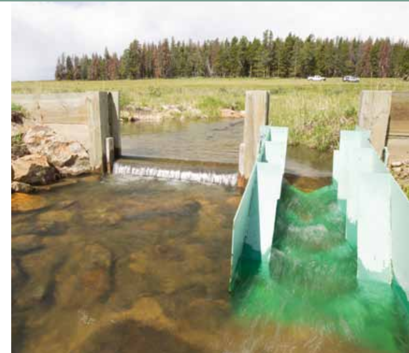
Using EQIP funding, this fish ladder installed in the Big Hole Valley of southwest Montana benefits arctic grayling. Farm Bill funding for projects like this helped preclude the need to list the fish under the Endangered Species Act in 2014. Photo by U.S. Fish and Wildlife Service.
